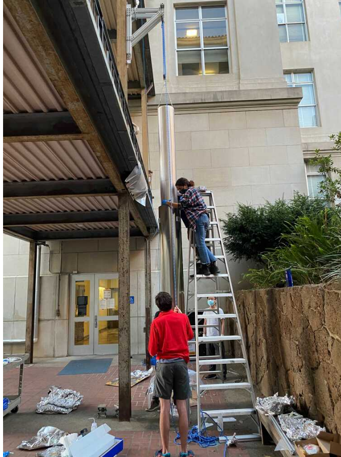
Figure 4.12: In case you ever doubted the strength of a single 1/4-20 bolt... The crane is attached to the I-beam with a single extreme strength 1/4-20 bolt from McMaster-Carr, though a thorlabs 1/4-20 bolt should have still had a large factor of safety.
